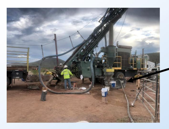
drill cuttings flow from the drill bit back up an inner tube into a cyclone then a splitter and a sample is collected for assay every 5 feet
